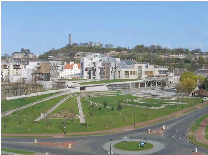
Figure 1: The new Scottish Parliament Building at Holyrood, Scotland designed by the Catalan architect Enric Miralles and opened in October 2004 1
