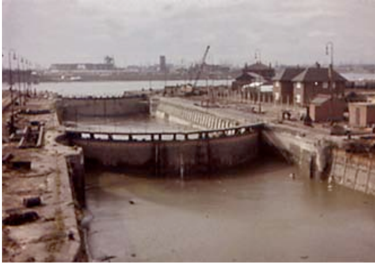
Figure 1: View of long-abandoned Western Entrance to RV docks prior to start of contract
