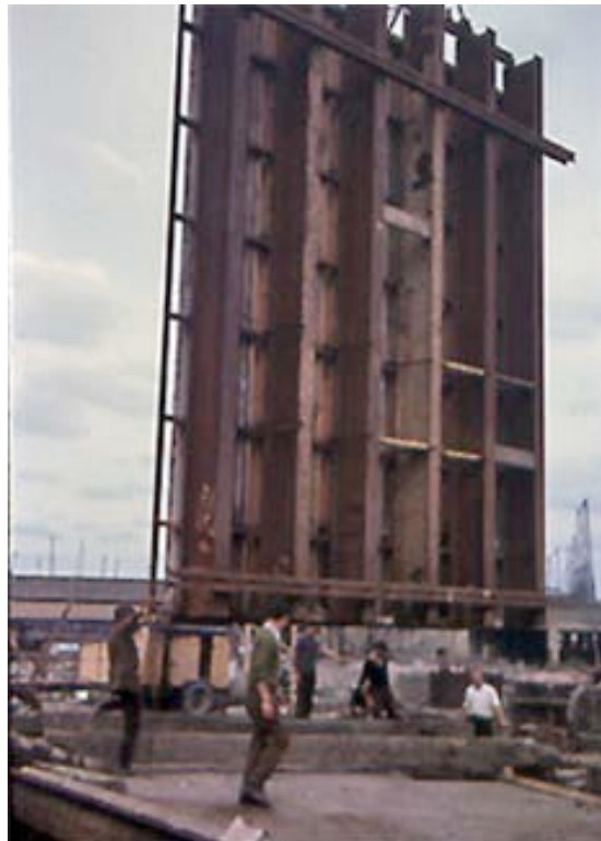
Figure 4: Lifting the "Big Form" into place.
