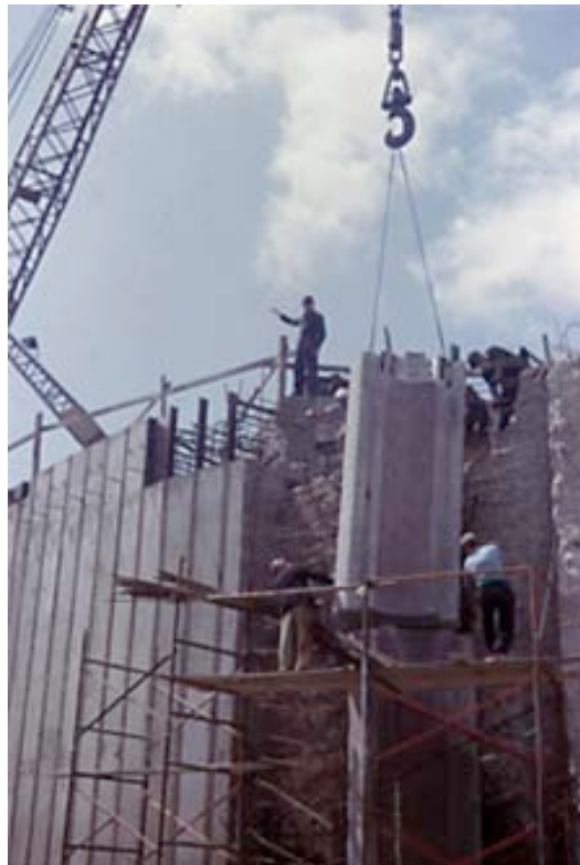
Figure 6: Lifting a precast concrete quoin unit into place
