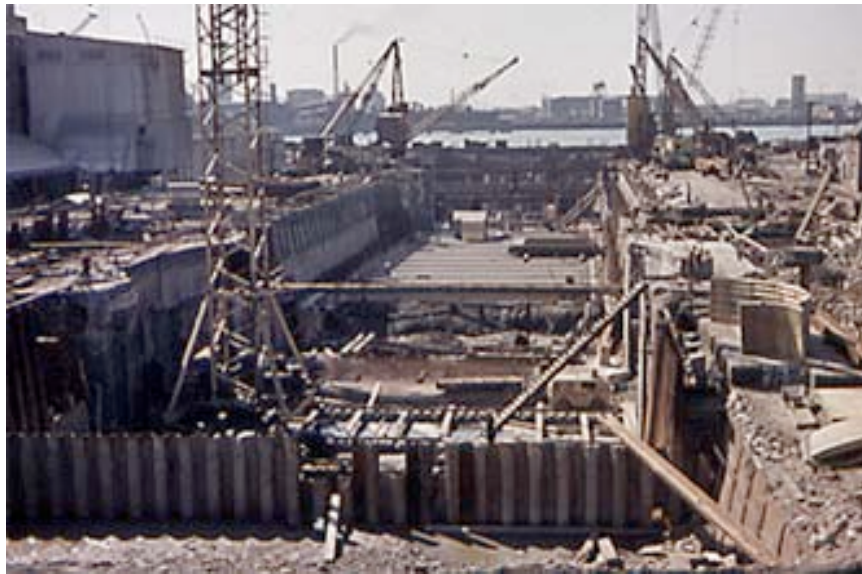
Figure 5: Excavation for the new lock floor well under way
