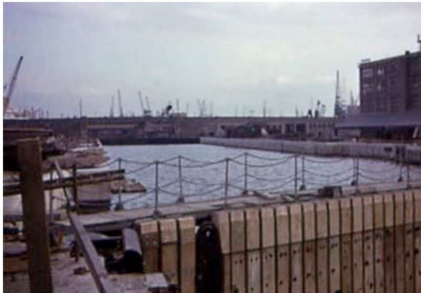
Figure 8: Finished lock filled to brim and under test.
