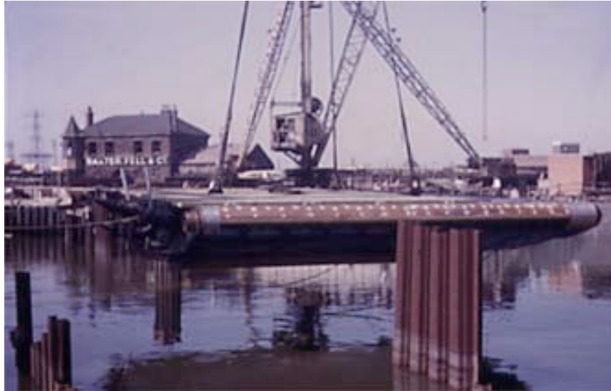
Figure 7: Lifting the 120-ton lock gate leaf into position.
