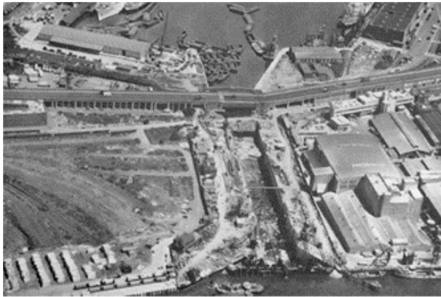
Figure 9: Aerial view of site at high tide in the river Thames during the peak construction period
