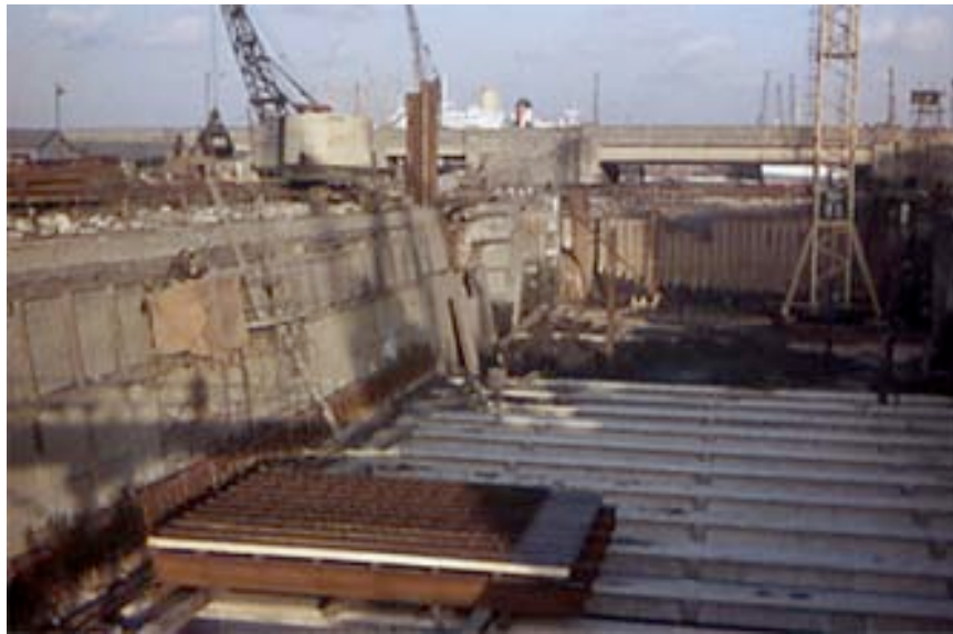
Figure 3: The dewatered lock and support to the aging walls
